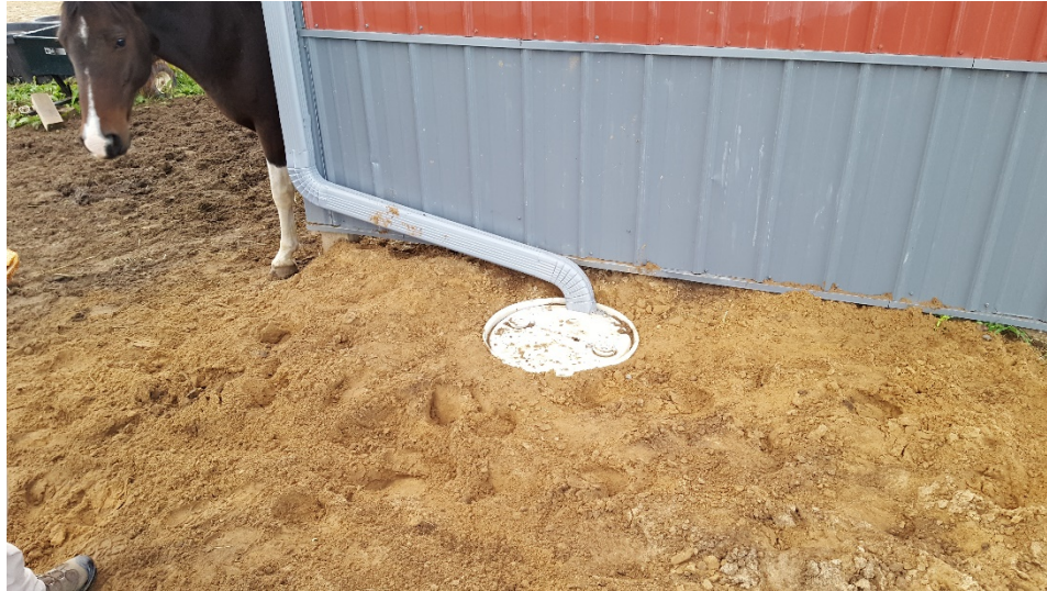
Figure 3: French drain stormwater BMP installed in a horse pasture, 2017.
