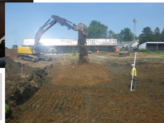
Picture right: The installation of the settling basin.
