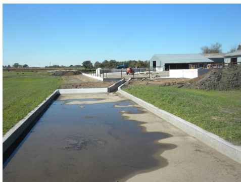
Pictured above is a manure pit and stacking slab that was installed for a dairy farm operation in Little Rock Lake watershed.
