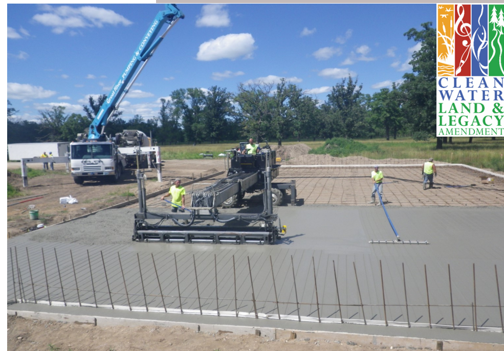
Pictured above: A before picture of the feedlot. Pictured below: The pouring of the stacking slab during construction.
